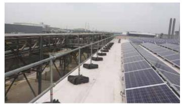
**KeeGuard® Premium** guardrail can also be used in combination with standard **KeeGuard®** where the counterbalance will not fit in with existing roof equipment.
