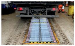
Note A & B Cover is deployed to prevent any fall into the pit. Make a formal weekly check of the condition of the cover.
